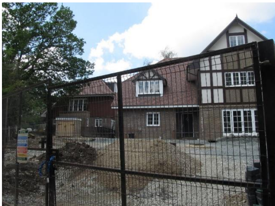
2 61 The Avenue under construction comprising flats disguised as houses
