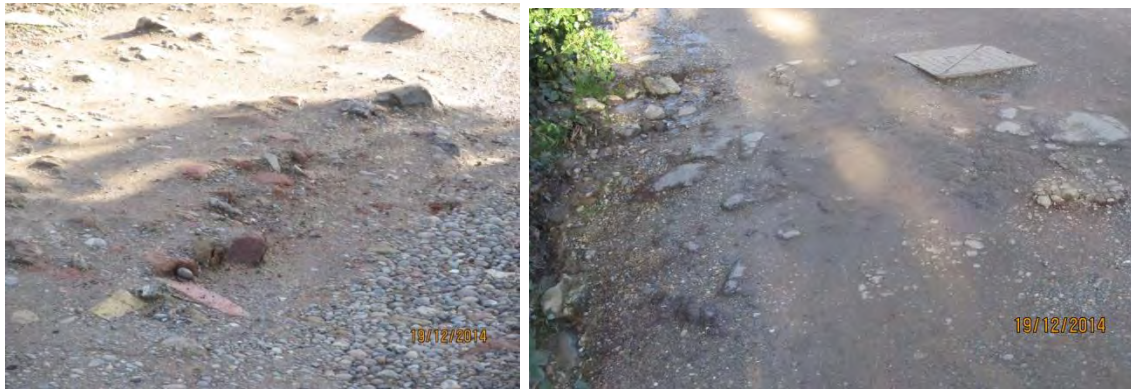
Figure 1 Typical road surface
