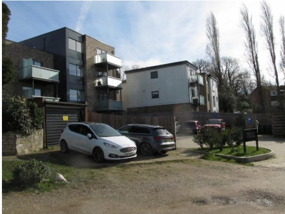
Above: clearly no fence on front boundary
