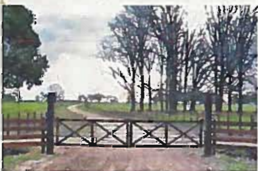
Timber entrance gates + fencing
