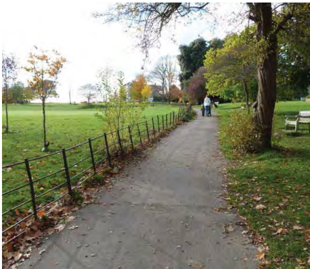
(e) Footpath lined with estate rail fence.
