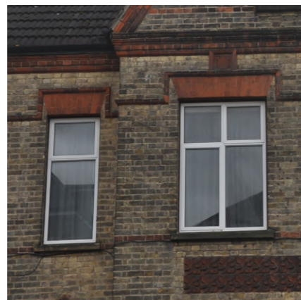
Detailing to highlight horizontal datums
