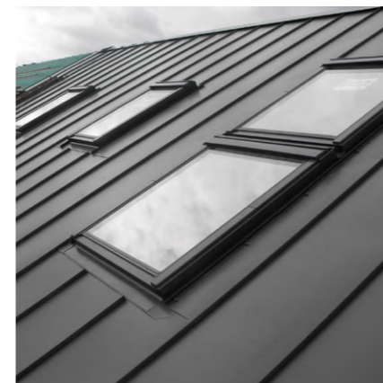
Rooflights within zinc standing seam roof
