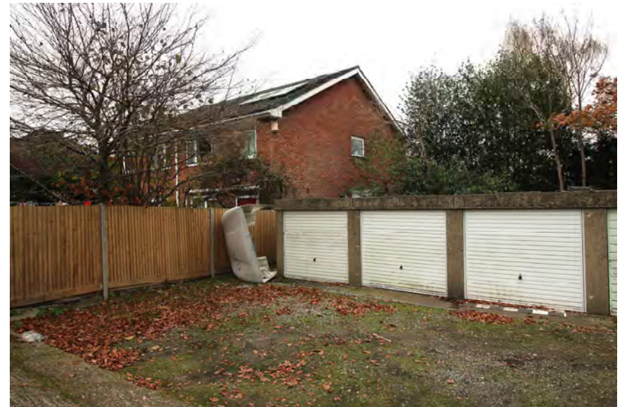
VIEW OF GARAGES SITE LOOKING NORTH WEST
