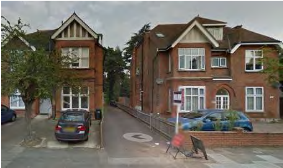
ACCESS LANE FROM HIGHLAND ROAD
