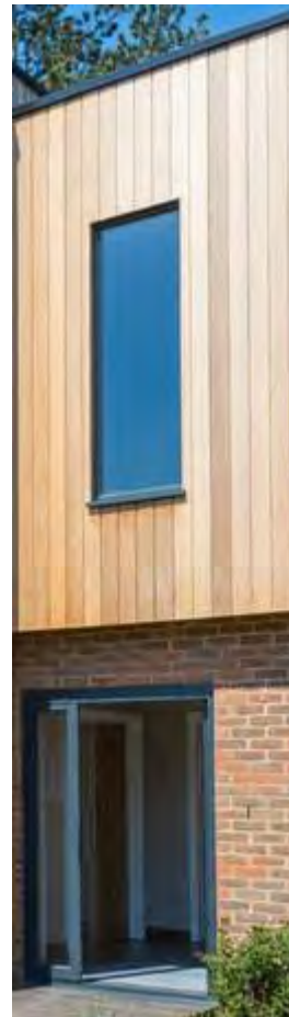
EXAMPLE OF: RED BRICK ON LOWER WALLS CEDAR BOARDING ABOVE ALUMINIUM FRAMED DOORS AND WINDOWS
