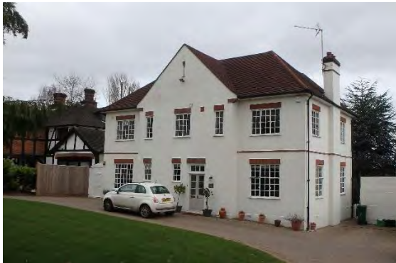
14 Downs Hill showing pitched and hipped roof with feature gable and white rendered finish
