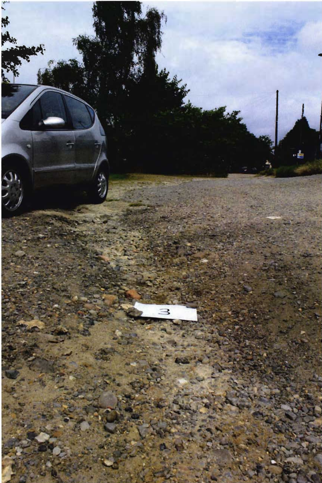
Picture 8: Item 3 shows erosion and an uneven road surface.
