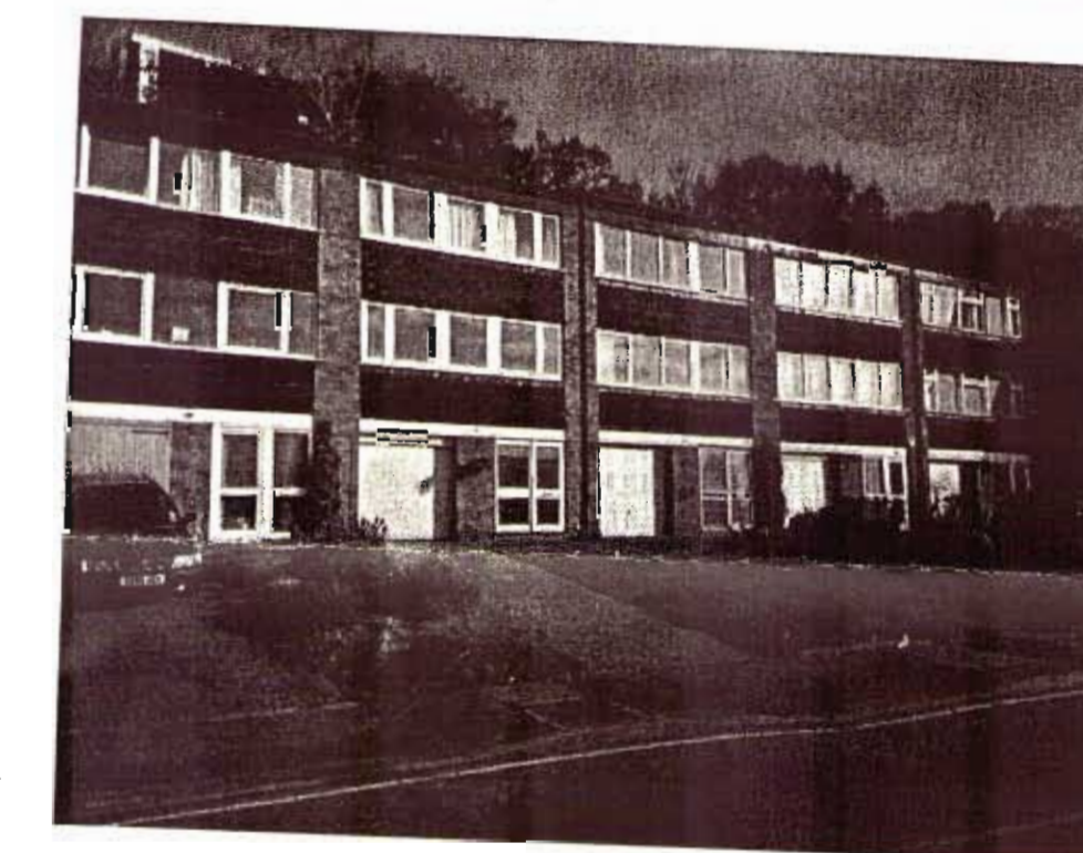
Examples of three / four storey dwellings on Madeira Avenue
