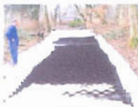
CellWeb during installation
