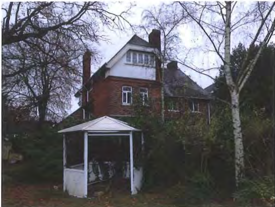
Rear of 4 & 4a Oaklands Road
