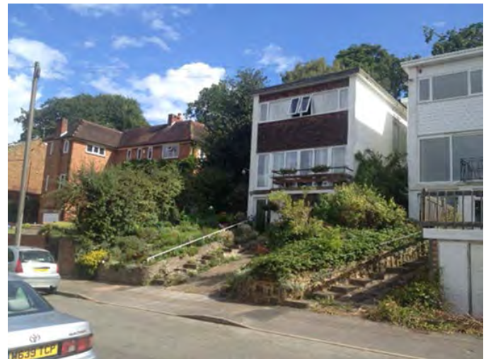
No 98 3 storey and No. 96 three storey with single garage below
